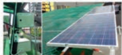
Figure 3: Installation of Solar Panel, Battery and Sensor to Car Park Structure
